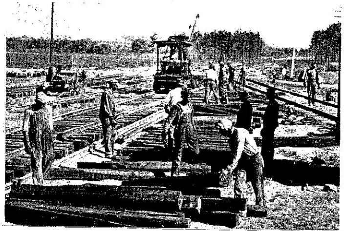
Track-laying on the L&N in Robertsdale, Ala. 1941. Apart from porter, track labourer was the chief occupation for blacks on Southern railroads in the first part of this century.
